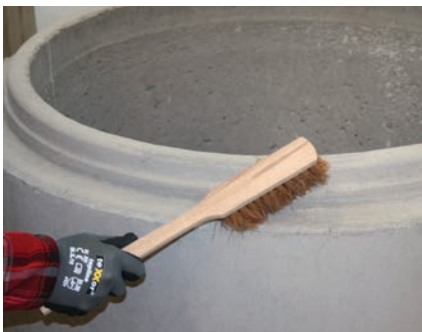
Image 4: Cleaning the connecting surface
