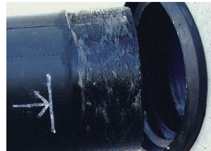
Image 8: Establishing the pipe connections
