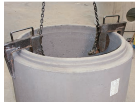
Image 3: Shaft suspension with claws
