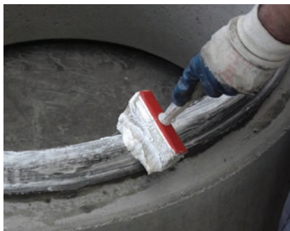
Image 5: Applying the lubricant
