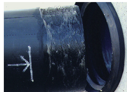
Figure 8: Creating the pipe connections
