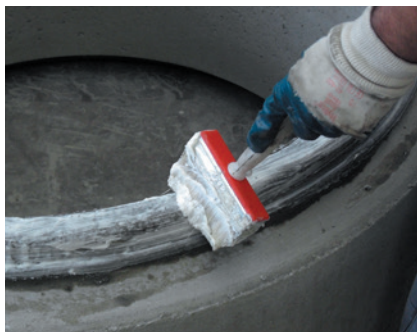
Figure 5: Applying the lubricant
