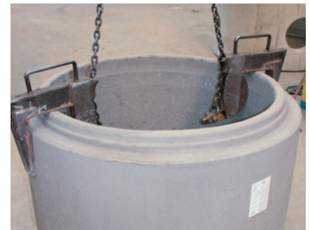
Figure 3: Shaft suspension gear with claws
