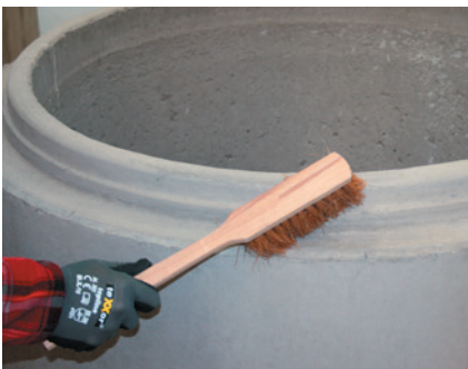
Figure 4: Cleaning the connecting surfaces
